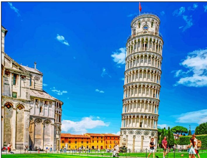
Leaning Tower of Pisa
