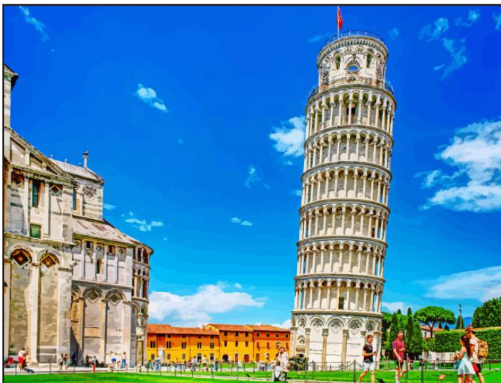
Leaning Tower of Pisa
